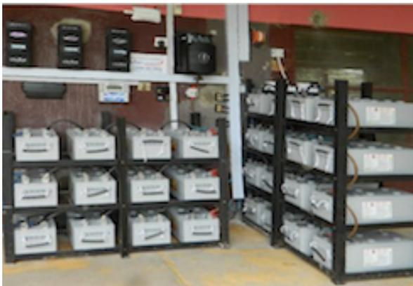
Deka Gel Batteries Used in the System
