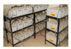
standard AC wiring and lights and drive them from small solar farms located every few kilometers along the roadway? His first "solar bunker" design was installed in March 2013 to supply 2.6 km of roadway in Plateau state. 18 kW of solar array feed Deka gel batteries and Outback inverters, which light 61 LED street light fixtures, for 12 hours per day. The total load is about 5kW and the system has been running for 4.5
