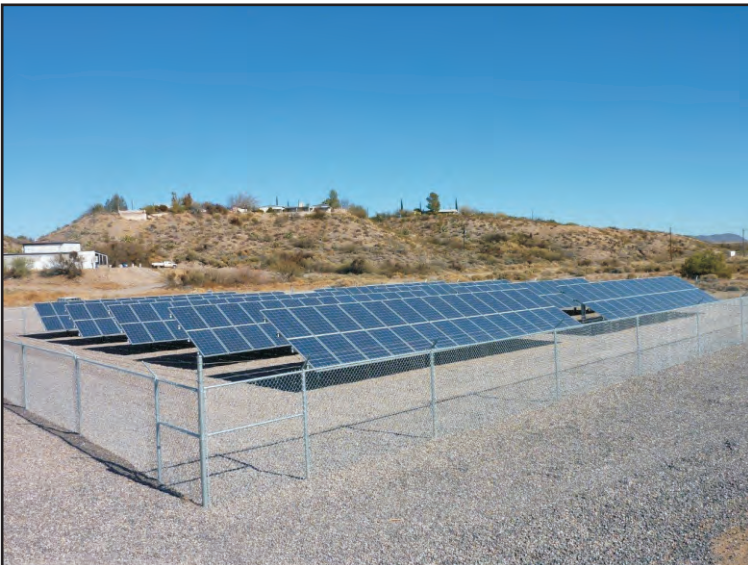
60 kW Photovoltaic Array
